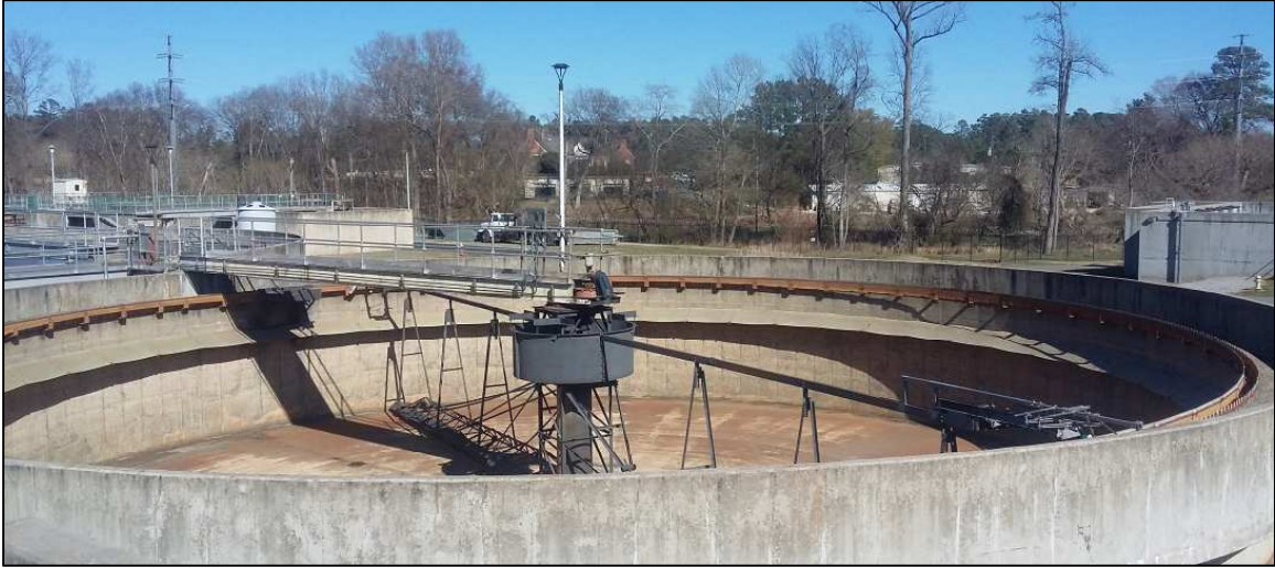
Photo 1: Envirex clarifier not in operation
