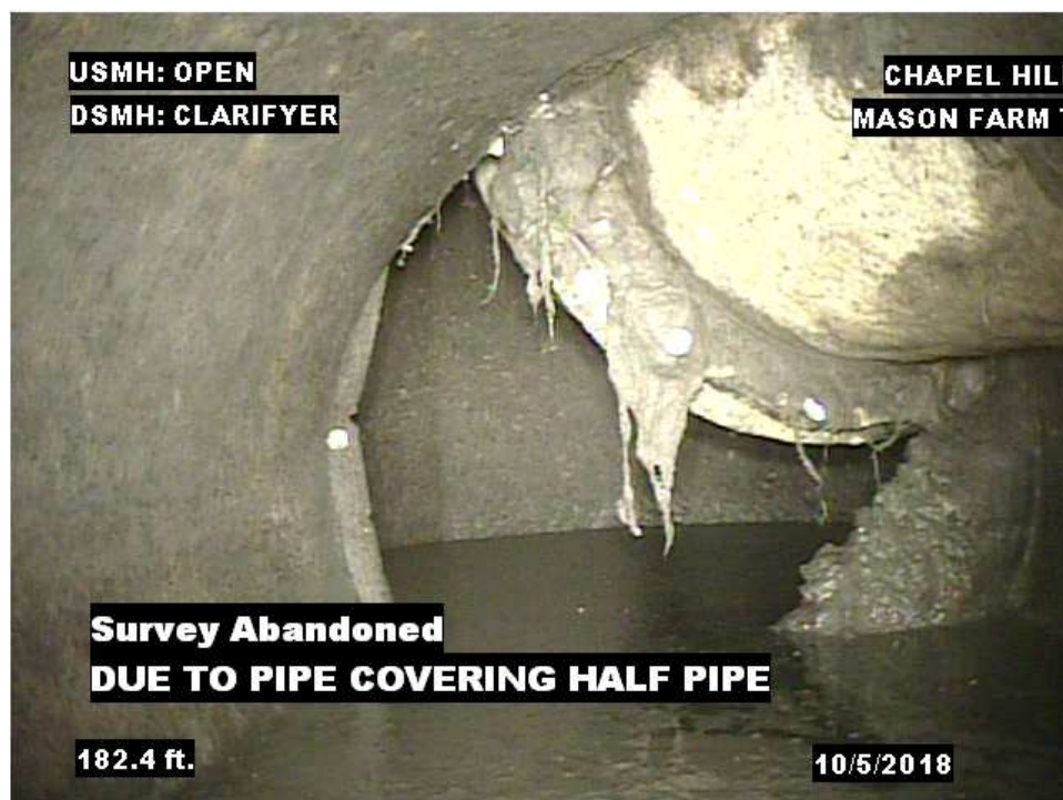
Figure 2-1: Clarifier 1 Pipe Survey
