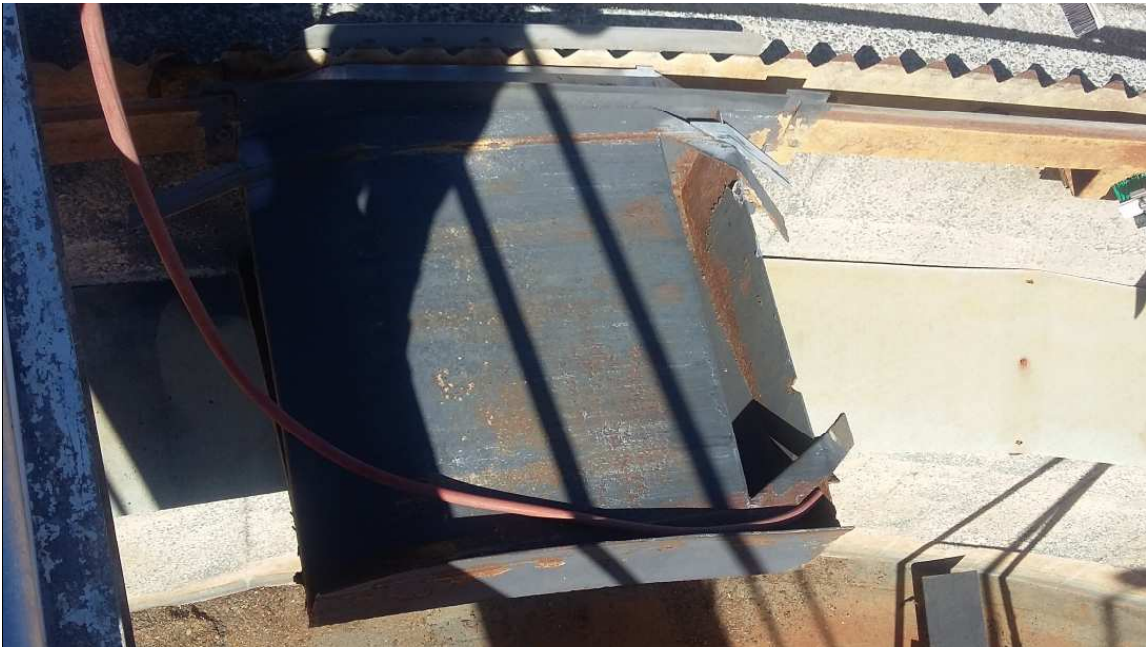
Photo 5: The scum troughs of both Envirex clarifiers are in a poor shape. Manual hoses are needed to complete flushing of the scum.
