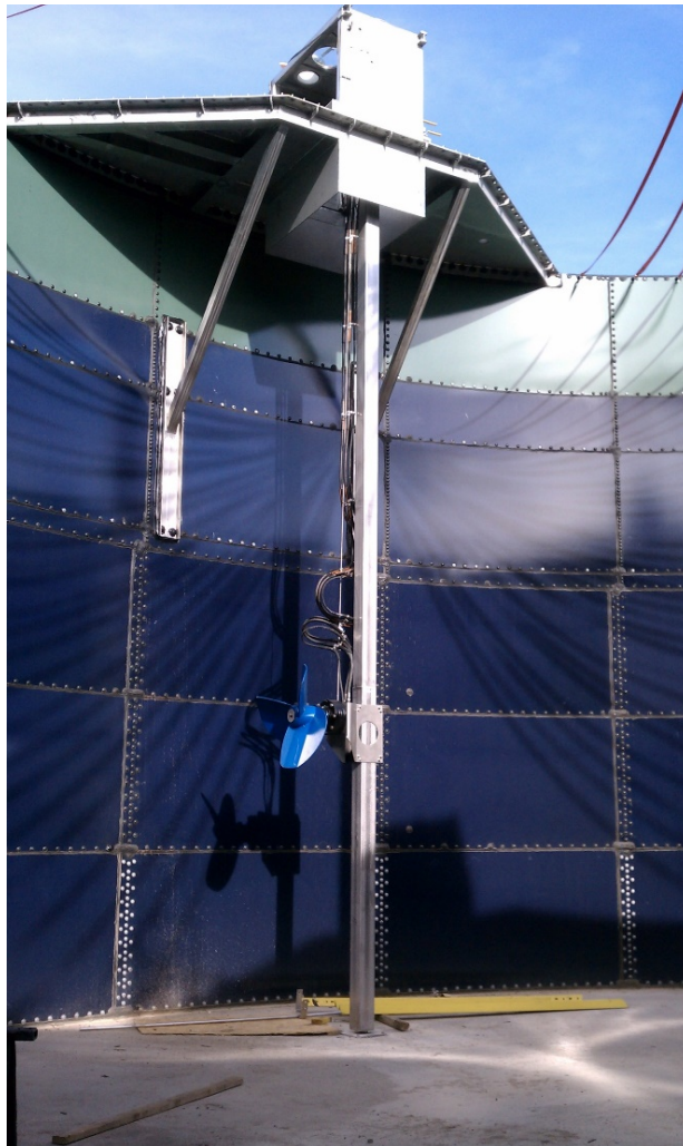
Figure 14. Example Installation of Anaergia Impeller Mixer
