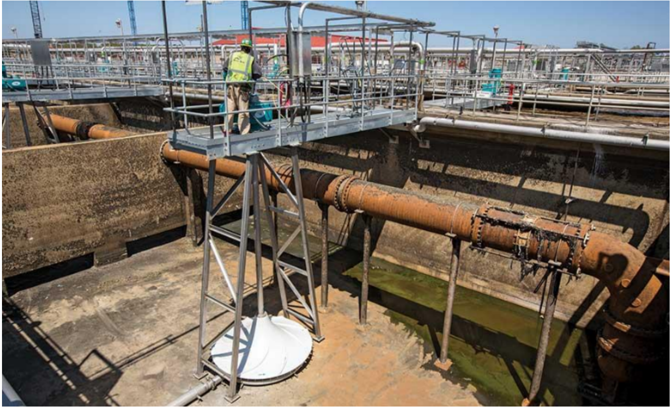
Figure 3. Hyperbolic Mixing with Tower Supported Platform (Basis of CDM Smith Conceptual Design)
