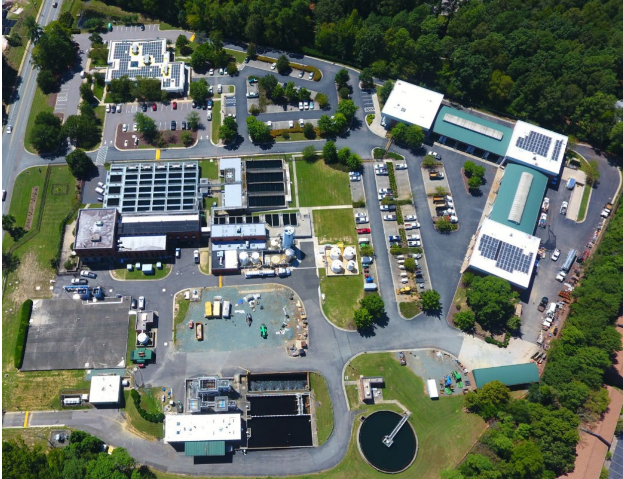
Jones Ferry Road Administrative Facilities and Water Treatment Plant
